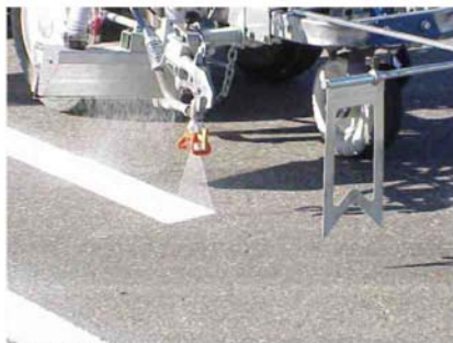
Figure13-c: Wind blew most of these beads South
