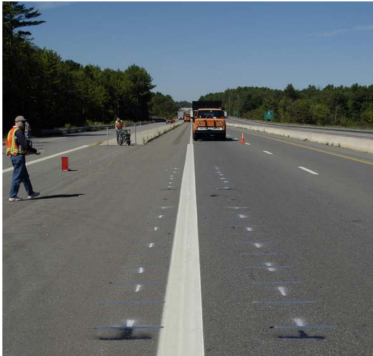
Figure 12: Epping Test Site, Just Prior to Paint Application.
